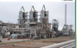
The Gas To Liquids Refinery (GTLR) is offline and undergoing currently preservation maintenance. The proposed project entails the reinstatement of the Mossel Bav Production Assets which includes the GTL-Refinery (Liquids Section) in the earliest possible time at minimum costs, following suspension of production in 2020 due to feedstock challenges.
