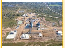
The Project is an expansion of South Africa's first and currently only onshore Production Right. It aims to increase the exploration, production and processing of natural gas and associated byproduct helium. The project entails a natural gas facility producing 12.5 million gigajoules of LNG per annum.
